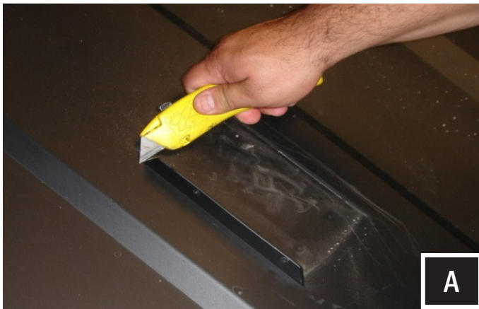
A. If the unit has a factory roof, you will need to first remove the roof and cut the dome light mounting flanges off using a utility knife.
